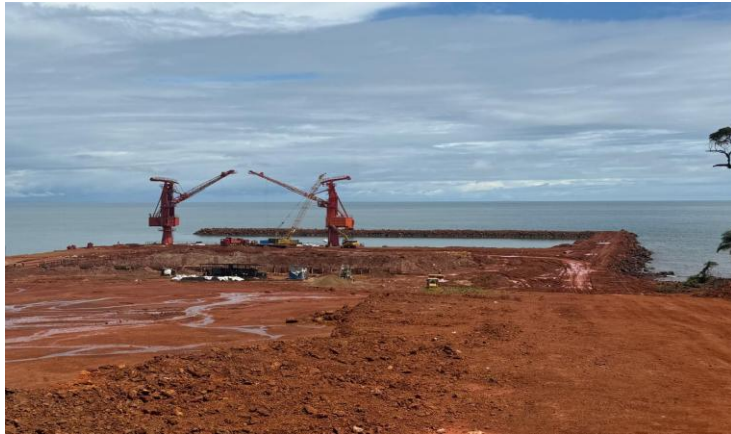
Cooperation Jetty construction Sole
